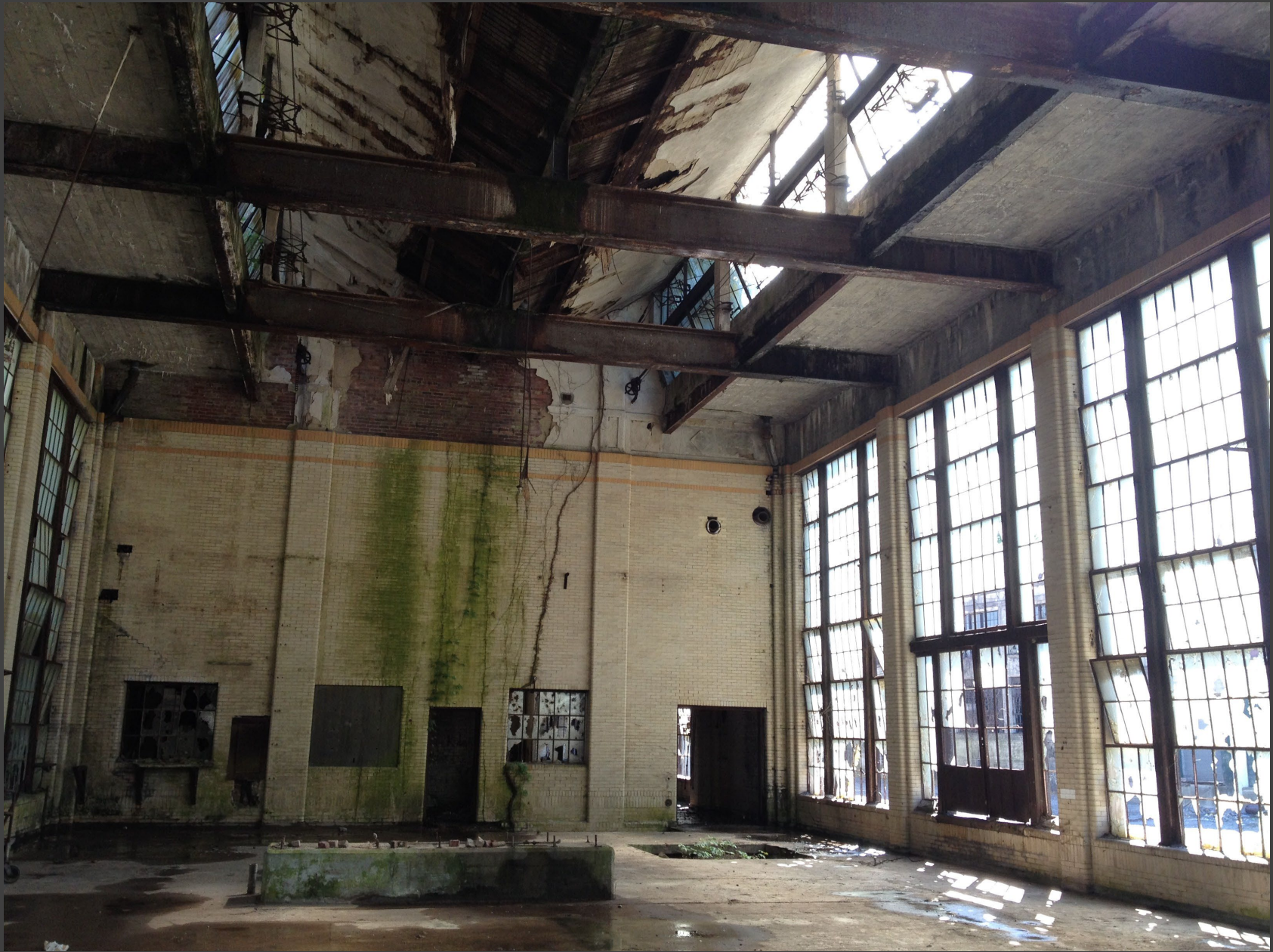
Peters Cartridge Factory Apartments - Before
